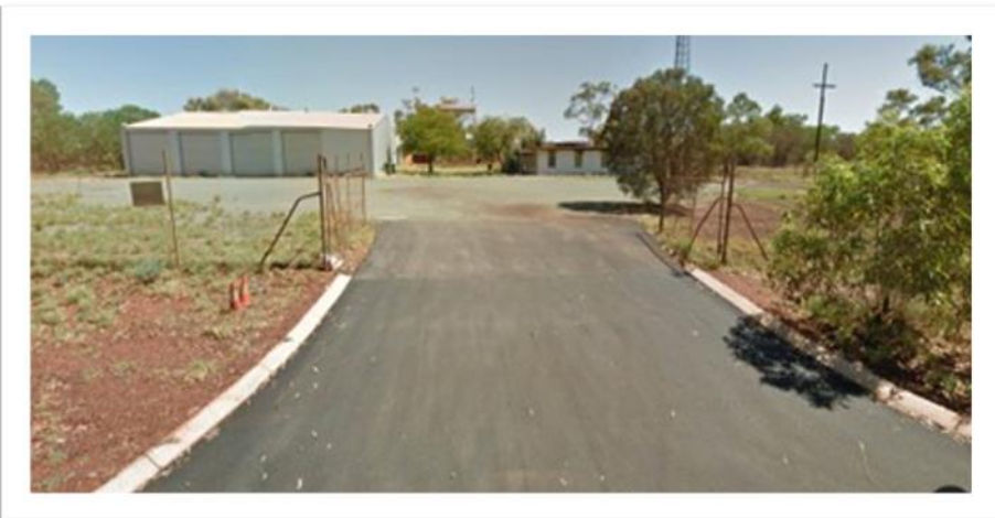
SES Newman Headquarters site before the new building was added.
