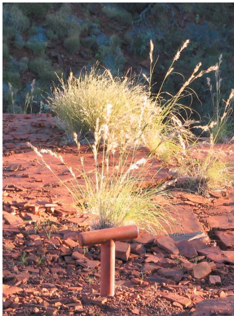
Pre-established manmade Anchor Point at top of gorge for rescues from Garden Pool.
